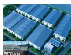
Dingxi Factory 甘肃定西
